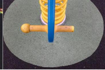
Finding: Stopper missing Action: New stopper required
