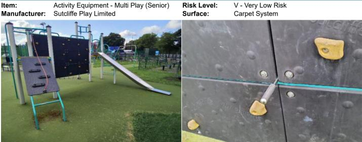
Finding: There is/are finger entrapment/s in the framework Action: Monitor - No remedial work recommended and the item fails to meet the requirements of BS EN 1176 Part 1 4.2.7.6 Entrapment of fingers
