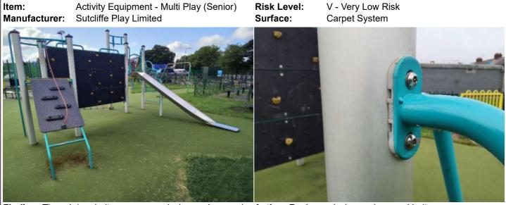
Finding: There is/are bolt cap covers missing or damaged Action: Replace missing or damaged bolt cap covers on the item
