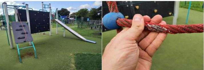
Finding: The ropes/nets are worn/damaged in places
