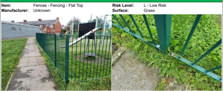
**Finding:** A number of fixings have worked loose around the **Action:** Secure all loose fixings fencing
