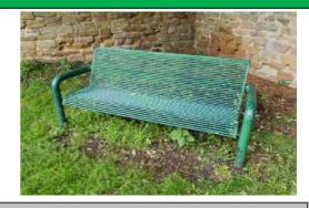
The paintwork on this item has been damaged or worn exposing the metal underneath which is rusting / corroding - in wet conditions - Reinstate the surface Treat affected areas and repaint
