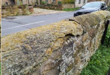
Finding: The masonry is loose, degrading or damaged
