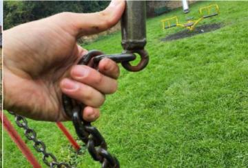
**Finding:** There is some notable evidence of wear to the anti **Action:** Monitor for any further deterioration and replace wrap bars when 40% worn
