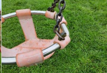
Finding: The connecting links are not seated correctly
