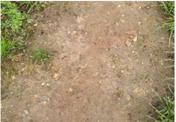
**Finding:** The grass has eroded within the impact area of the **Action:** Reinstate the grass or provide an all weather equipment exposing rocks and rubble and may not provide surface the necessary impact attenuating properties for the equipment fall height; the surface may also be slippery in wet weather
