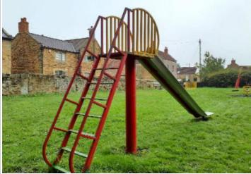
**Finding:** The surfacing dimensions are short and do not meet with the requirements of the current applicable standard (1.76m required / approximately 1.2m provided)
