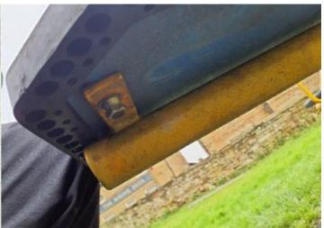
Finding: Shear nuts have not been fully tightened and are Action: Tighten heads on nuts to shear off and secure still present on fixings
