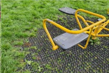
**Finding:** Parts of the steel structure protrude beyond the protected elements of the seat and fail to meet the requirements of BS EN 1176 Part 5
